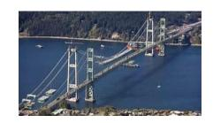
8iEngineers need to consider loads when building structures. Loads are weights and forces that a structure must withstand. The dead load of a structure is the weight of the structure itself. The dead load of the bridge, for example, includes beams, cables and the deck. The live load of a structure is the weight that is added to the structure, including people, cars and the wind.
