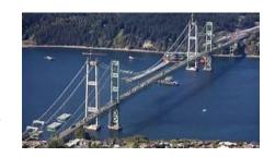
Engineers need to consider loads when building structures. Loads are weights and forces that a structure must withstand. The dead load of a structure is the weight of the structure itself. The dead load of the bridge, for example, includes beams, cables and the deck. The live load of a structure is the weight that is added to the structure, including people, cars and the wind.
